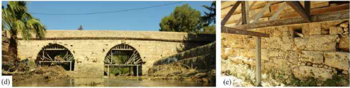
Figure 2: (a) Rhodes Island in Greece and location of the Roman bridge, (b) top view of the Roman bridge, (c) and (d) Roman bridge from different views, and (e) openings in the central pier with erosion.
